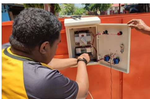
Gambar 3. Instalasi kontrol panel
